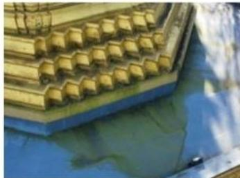
P05 Gold paint failing collecting on flat roof
